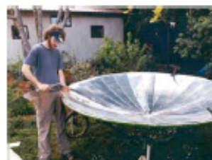
HSU student riveting aluminum to dish.
